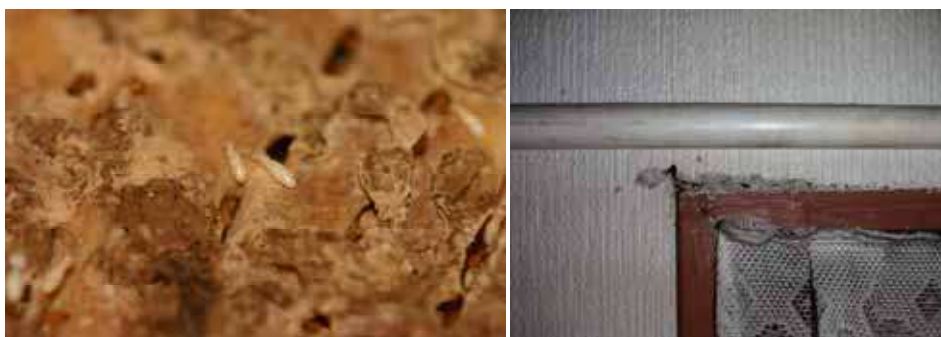
Fig. 1. Left: workers and soldiers of Coptotermes formosanus in their nest. Right: Damage on a residential structure caused by foraging termites of C. formosanus
