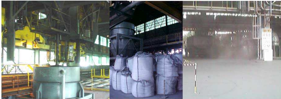
Fig. 16. Dust discharging at Albras bake furnace, implemented solution in the left side, in the center discharge of dust in big bags, free falling of dust in truck in the right - source: Albras Alumínio Brasileiro SA.
