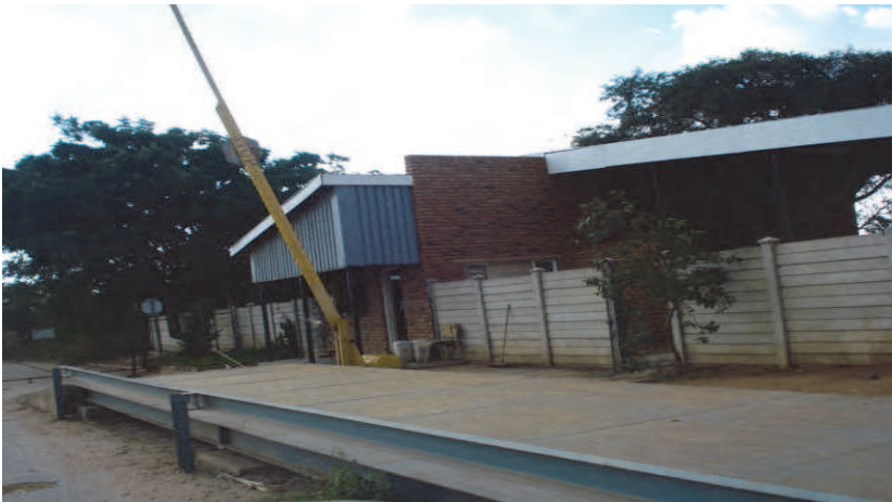
Fig. 8. Weighing bridge at the entrance of the Polokwane landfill site.
