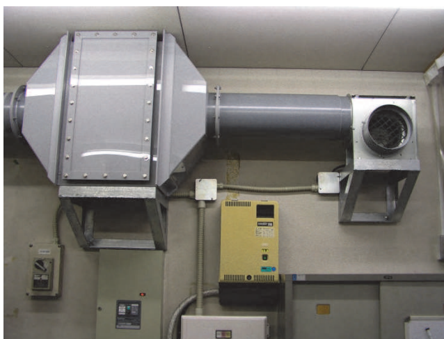
Fig. 6. Centrifugal blower (right), charcoal filter housing (left) and humidifier (center).
