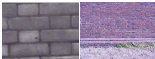
Fig. 18. Brick Wall Infrared (left) and Visible (right) Images.
