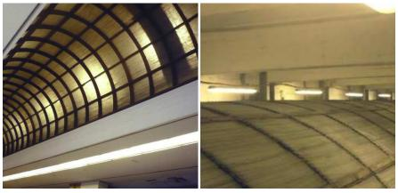
Fig. 7. Actual condition of the vault and back lighting vault (luminaries with fluorescent lamp)
