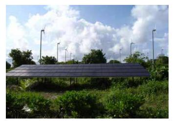
Fig. 13. Micro-wind farm and photovoltaic panels as installed in the Uligam island
