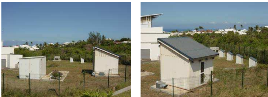
Fig. 6 & 7. The experimental platform and the test cells
