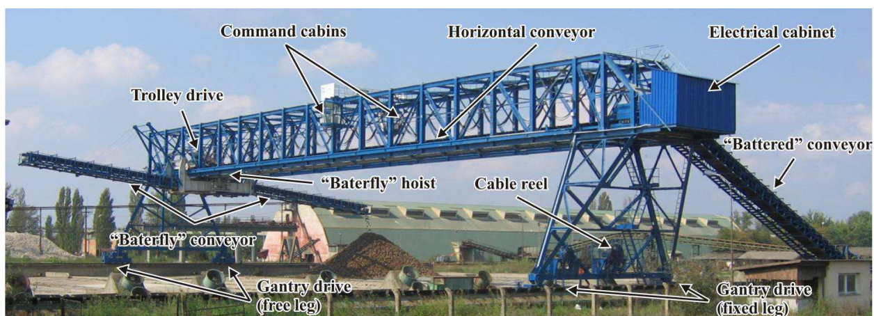
Fig. 18. Gantry crane with indicated drives.
