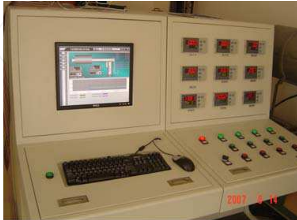
Fig. 12. Monitor equipment of heat pipe technology
