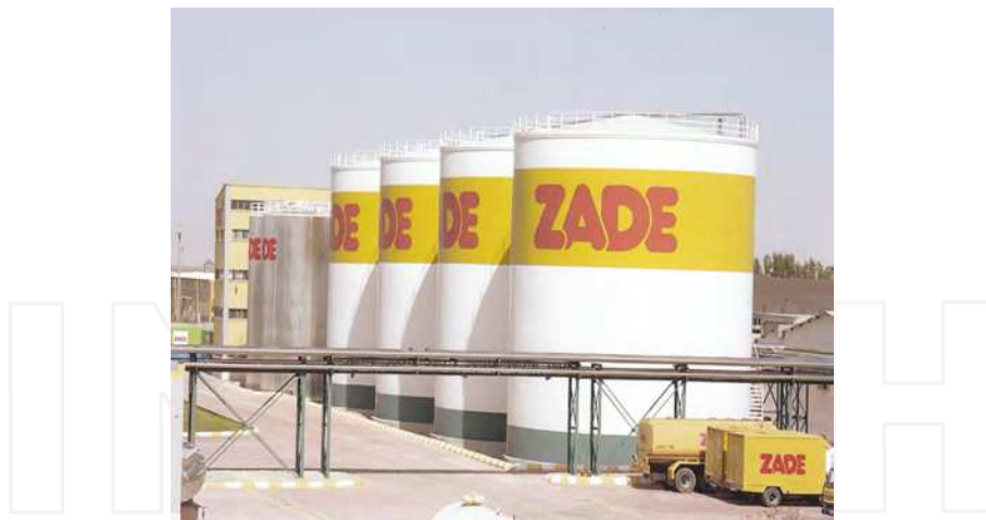
Fig. 5. Crude Vegetable Oil Silos
