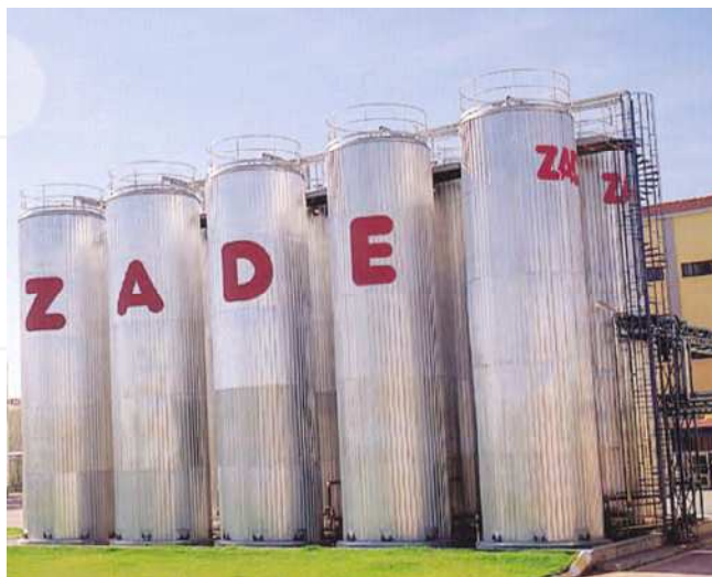
Fig. 11. Refined Oil Silos
